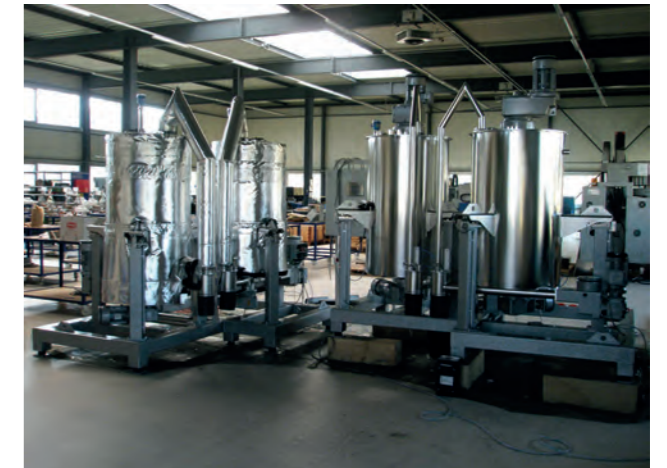
Battery production feeding systems completely insulated
